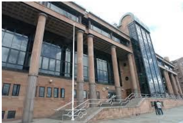
Newcastle Crown Court
