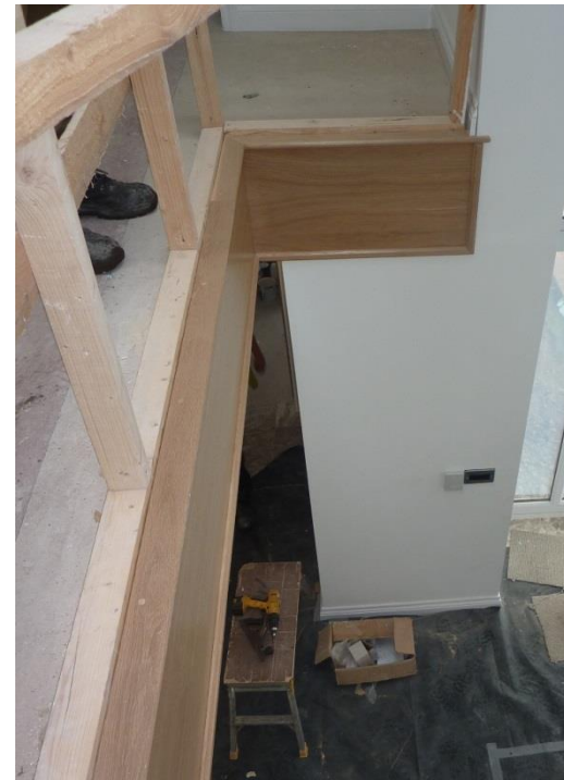
This photo shows the landing AFTER a guard rail had been fitted
